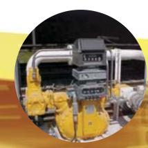
As accurate as filling station pumps, VTC's metered pumps are calibrated monthly and designed to be accurate to twenty five one-hundredths of a percent per gallon.
